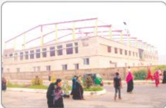
Outside view of Vancot Limited financed by SBL, Agrabad Branch, Chittagong.
